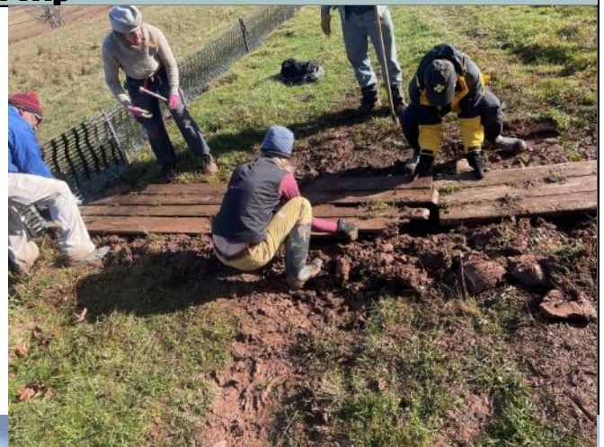
right PATC-STS workers attack a bridge photo by Chip Chase
